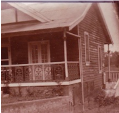
Illustration 12. Arthur’s ‘French flourishes’ - French doors from the bedrooms onto the front verandah and wrought iron fleur-de-lis panels enclosing the verandah.
