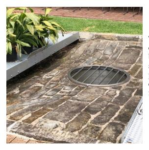
This is the latest reincarnation of the cistern in the courtyard of Carisbrook, thanks to lots of hard work by many. This huge underground sandstone-lined storage tank holds over 28,000 litres of crystal-clear pure water. Unlike other cisterns this water is collected from roof run off and then naturally filtered through the sandstone.
