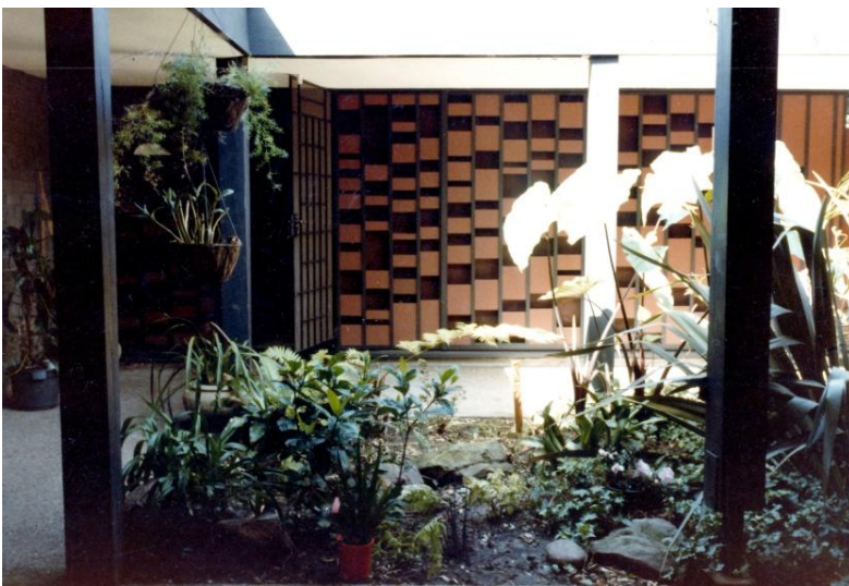
Gruzman's ornamental screen at the front door had deteriorated and was difficult to clean. The wall was restored with panels of opaque glass. Two skylights were added to the hall inside the entry which lit the area..
